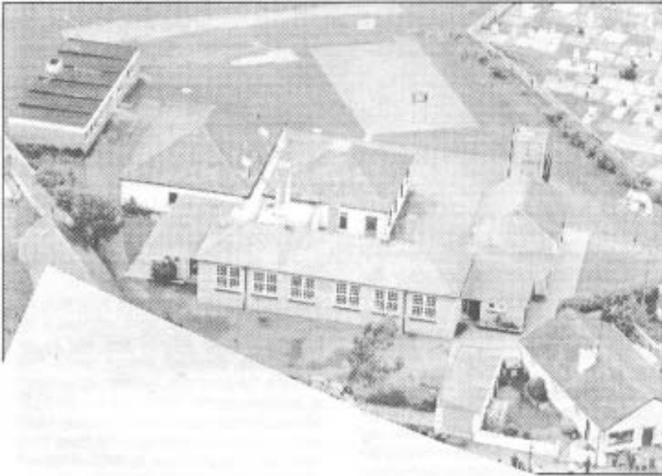
Aerial view of Tinryland NS
